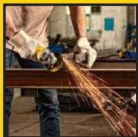
1 Cutting Rebar; Grinding Welding Lines Small Angle Grinder SG7100/SG5100
