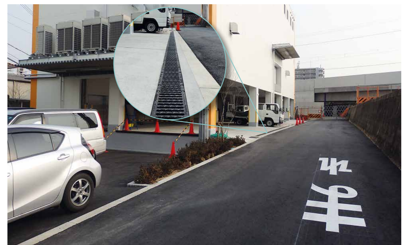
Sanwa Food Company - Office building, Osaka, Japan
